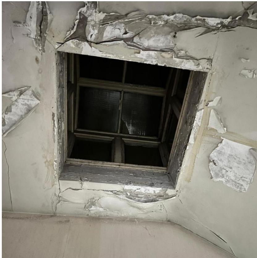
**Figure 48 – Photograph of inside of existing roof lantern. The lantern has been made weathertight and boarded up whilst the application is considered.**
